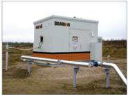
**WELLHEAD CONNECTION** Either hard pipe or flexible hose may be used.
